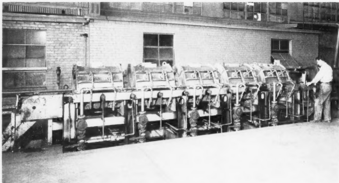
Line of barrel type furnaces, with quenching and conveying equipment, takes only one-fourth the space required for conventional bar annealing system
